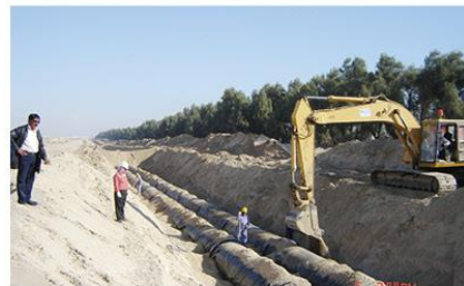
Jeddah DN1400 project, Saudi Arabia
