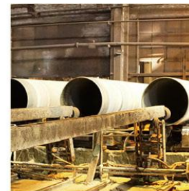
Cement lining grinding
