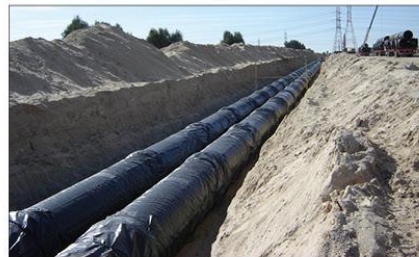
Kuwait SE100 DN1400 project
