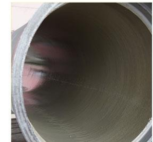
Cement mortar lining
